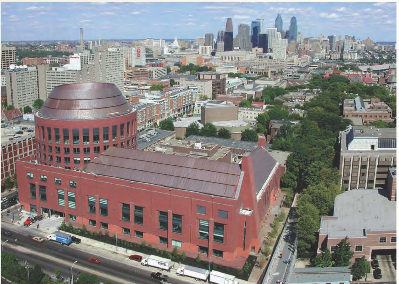
THE JON M. HUNTSMAN HALL, WHICH OPENED IN 2002, IS A $140 MILLION BUILDING AT THE WHARTON SCHOOL OF THE UNIVERSITY OF PENNSYLVANIA.
